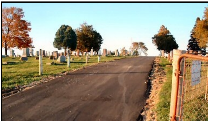
Blacktop going north on east side of the cemetery.
